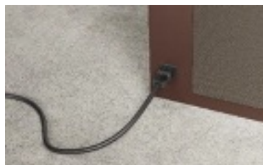
Illustration 2 - Power and data connection through column side
