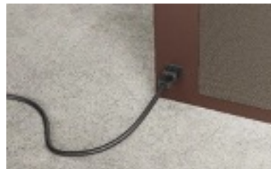
Illustration 2 - Power and data connection through column side
